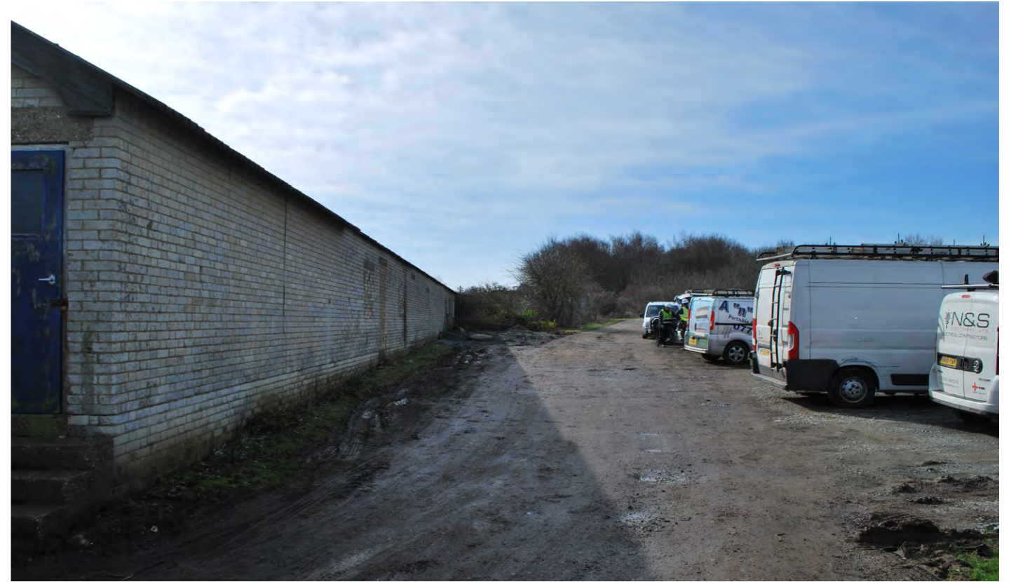
Former WWII ablutions block along airport boundary with the Innovation Centre
