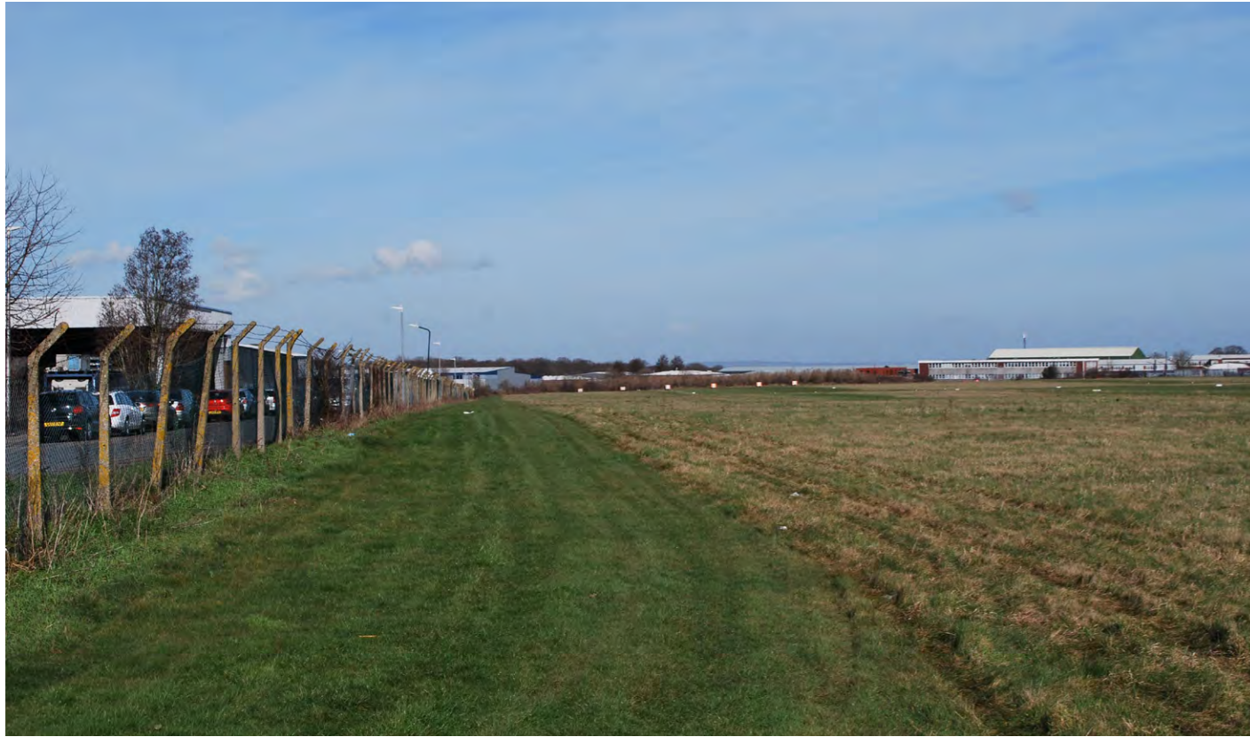
View looking north along the western boundary of Parcel 1
